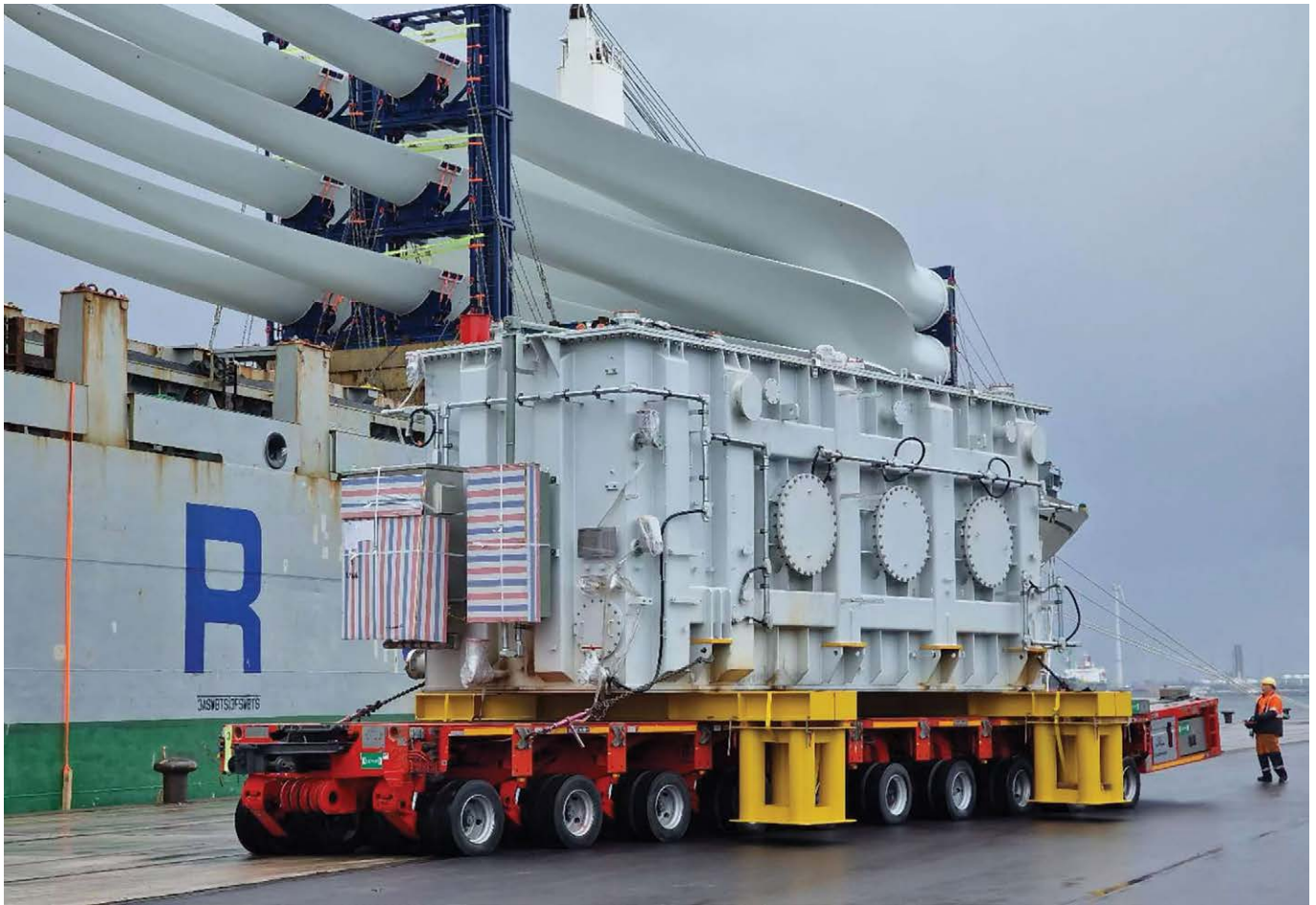
The first CHINT 400 kV transformer lands in Germany.
