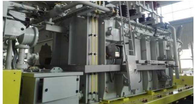
Ecuador 46kV Mobile Substation
